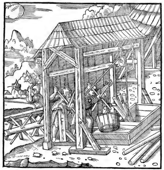
A-Windlass. B-Straight levers. C-Upright beams. D-Rope. E-Pulley. F-Timbers to be lowered.
